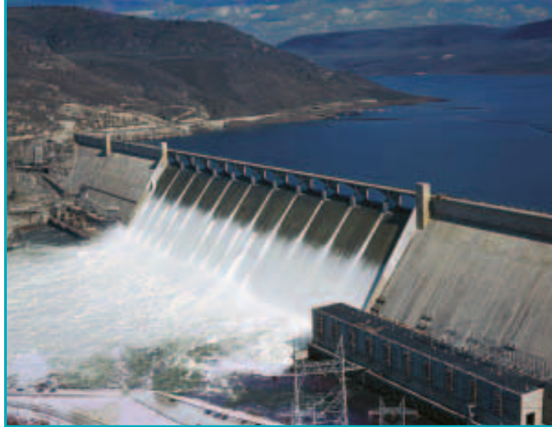
▲ Hydroelectric plants such as this one in Washington state produce about 10 percent of the power used in the United States.
