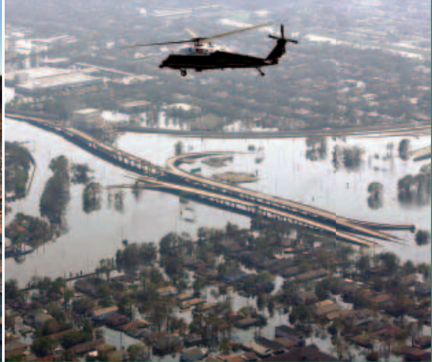
▲ Hurricane Katrina flooded much of the Gulf Coast, including New Orleans.
